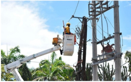
Power technician repairs a transformer.
